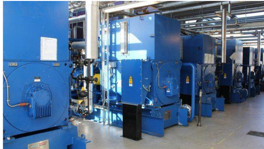
13.2 MW seawater heat pump (Oslo, 2011)
