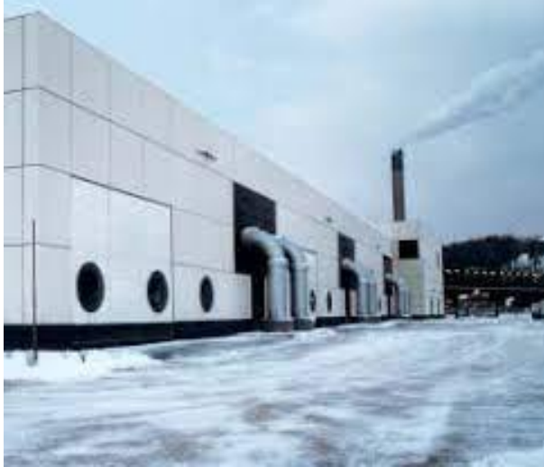
180 MW seawater heat pump (Stockholm, 1986)
