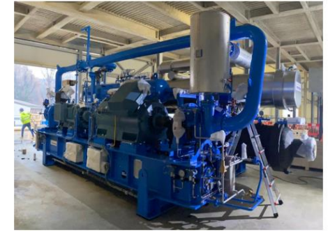
HP MM Salemi during erection (IT)
