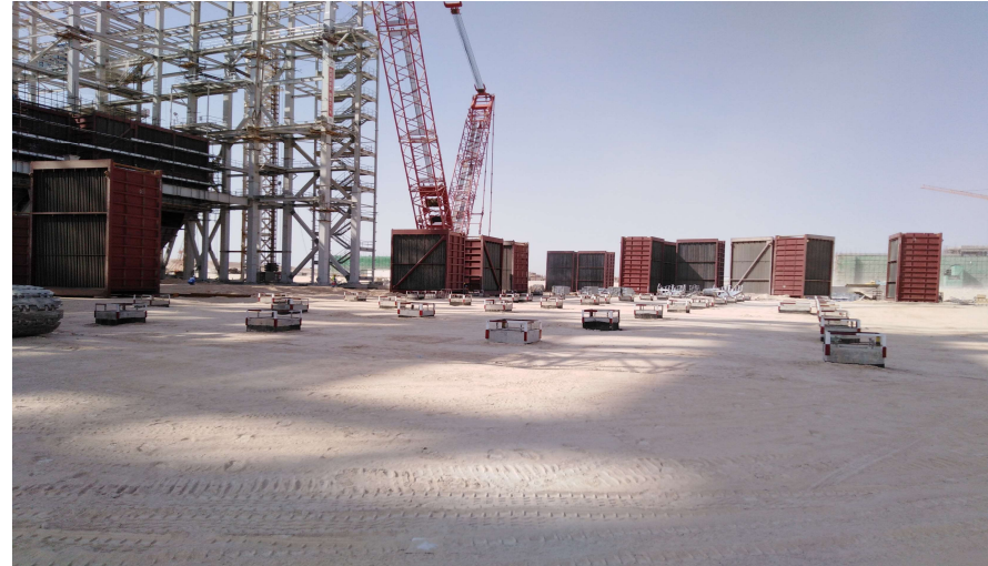
Unit 2 Boiler APH installation
