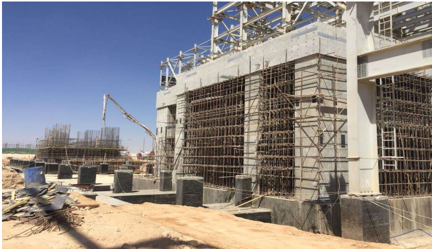
Unit 1 STG foundation works
