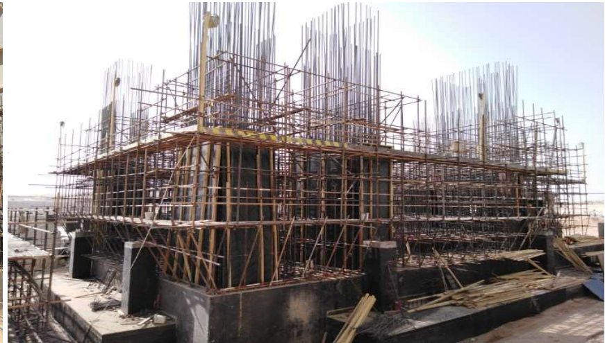
Unit 2 STG foundation works
