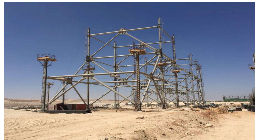
Unit 1 ACC steel structure installation in progress
