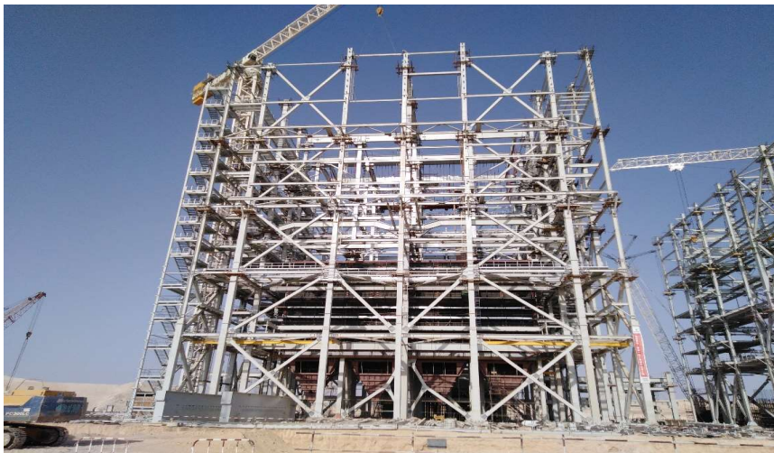
Unit 1 Boiler steel structure works
