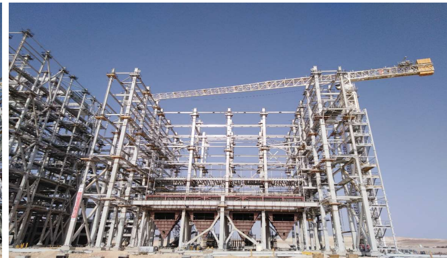
Unit 2 Boiler steel structure works
