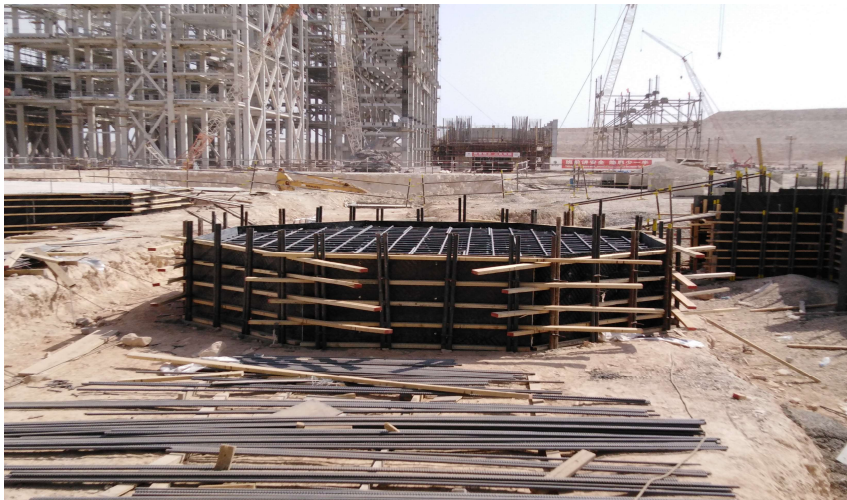
Water Tanks foundation works
