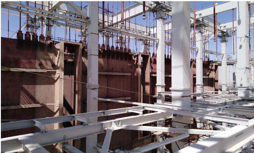
Unit 1 Boiler furnace water-walls installation
